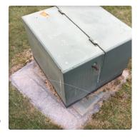
At least 3 feet of space on sides and behind the transformers are necessary to prevent them from overheating and causing a service interruption. Like all types of transformers, they need plenty of air circulation around them.
